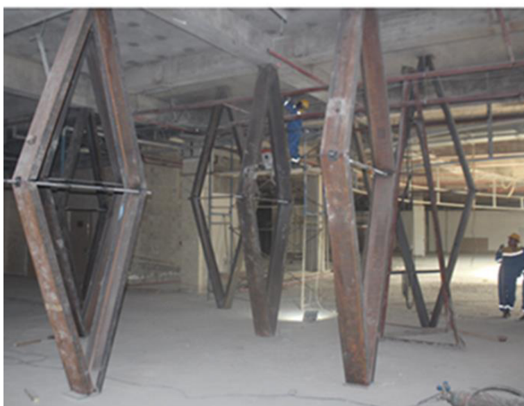
Figure 1 – Raising the floor with telescopic racks (author’s material)
