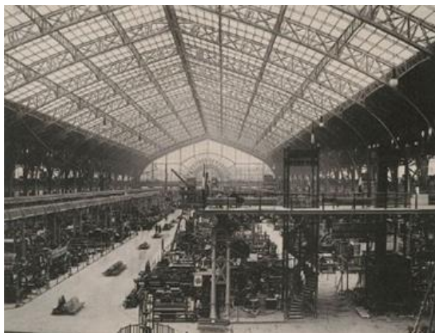
Figure 3 – Gallery of Machines, arch. Duther, Eng. Cotansen, Paris, France, 1889. View of the interior space
