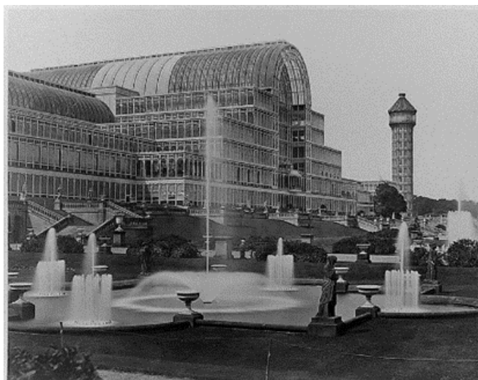
Figure 1 – Crystal Palace, arch. Joseph Paxton, UK, mid-19 th century. General view. A Dorling Kindersley book. Architecture. 1999 [4]
