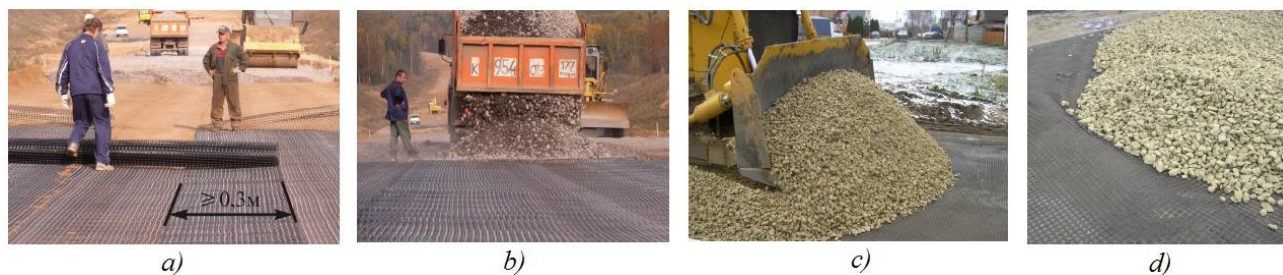
Figure 5 – Separate working operations when reinforcing road surfaces: a – laying a geogrid; b – filling the material of the supporting base; c – leveling the material according to the method «from yourself»; d – formation of a «wave» before the leveled layer [7]
