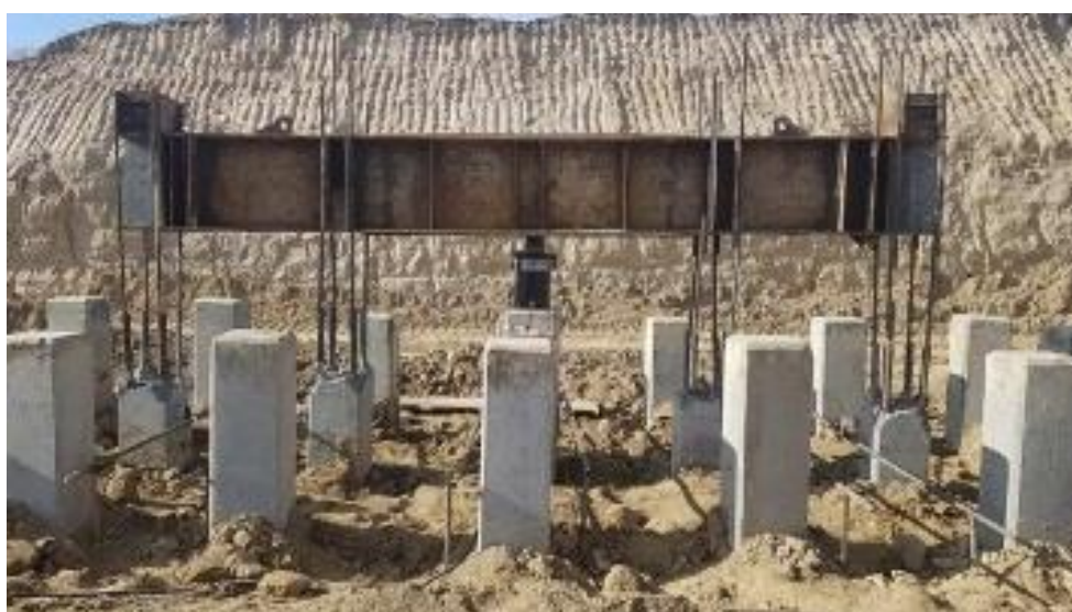
Figure 2 – General view of the measuring system of pile № 45 prepared for work.
