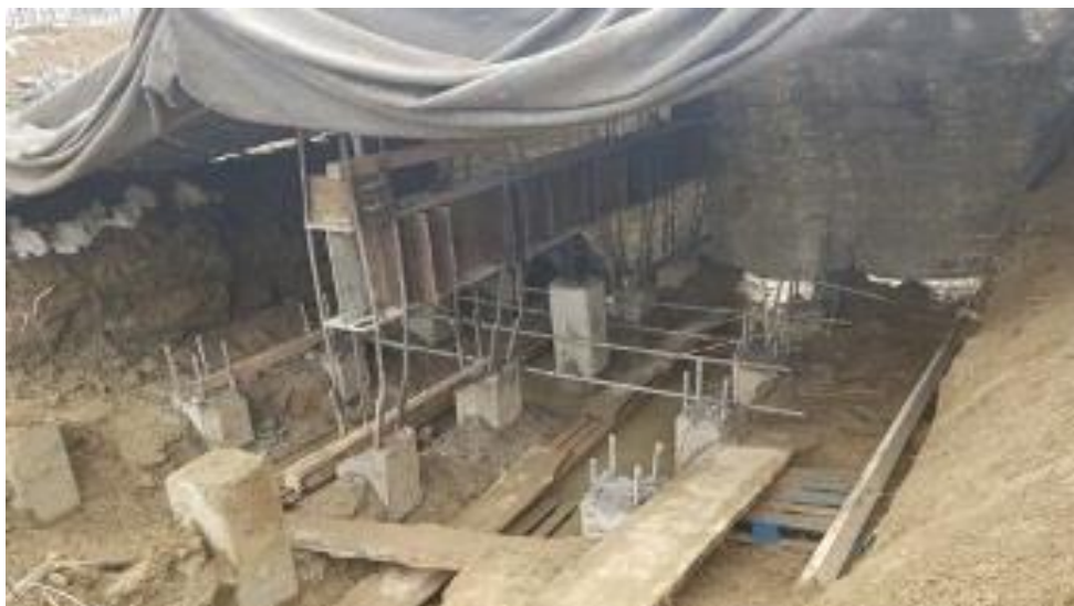
Figure 1 – General view of the measuring system of pile № 38 prepared for work.
