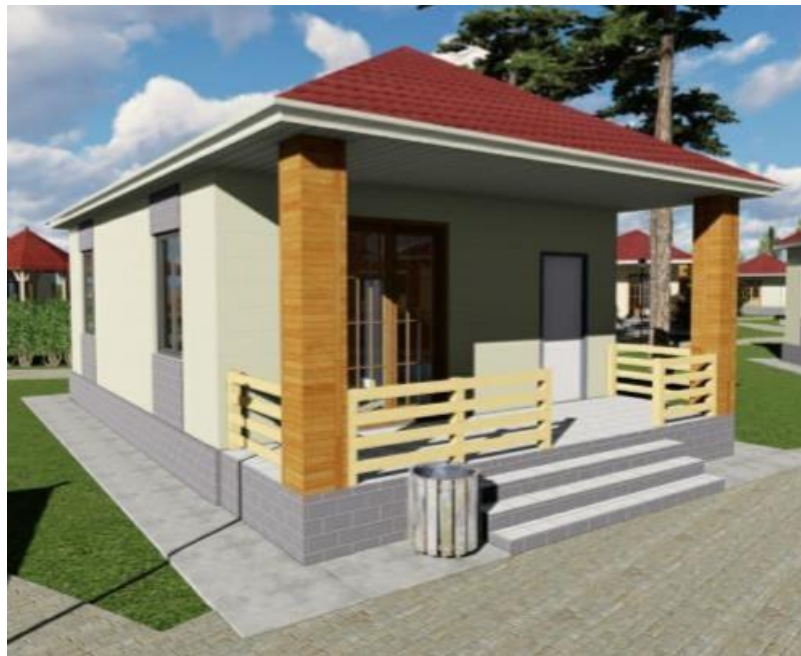
Figure 3 – Facade of a type 1 house
