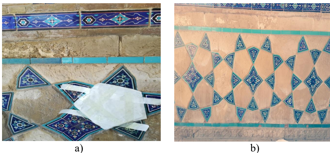
Figure 2 – Example of overlaying the compress (a) and the area of salt cleared with a compressor method using the solution of Trilon B (b) [author's material].
